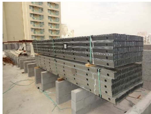
Figure 19 – Tracks and studs profiles stock placed outside the building without protection.
