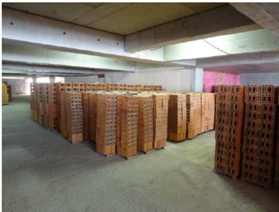
Figure 16 – Block stocks usually occupies a significant area inside the building to guarantee provision.
