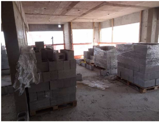
Figure 22 – Concrete blocks at the floor where masonry is just to be built.
