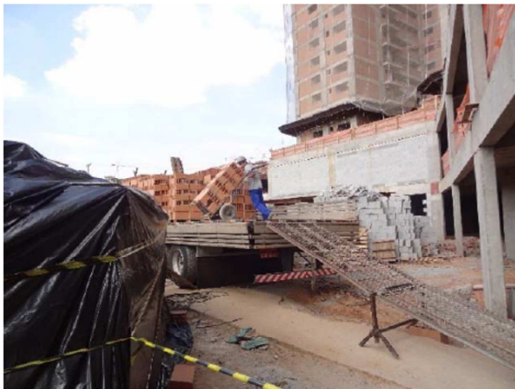
Figure 14 – Ceramic blocks are received at the construction site. General contractor manages acquisition and supply.
