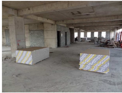
Figure 23 – Gypsum board at the floor where DW is just to be installed.
