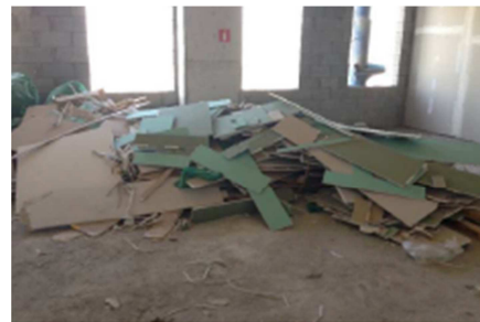
Figure 31 – Gypsum boards waste.
