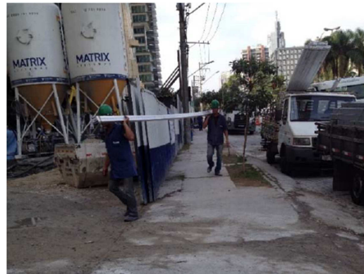
Figure 15 – DW studs profiles being delivered at the site. Supply and transportation is under installer control.
