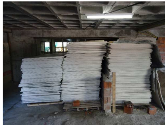
Figure 13 – Gypsum boards are also stocked inside the building but demands a smaller area
