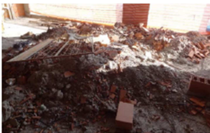
Figure 30 – Ceramic block and mortar waste.
